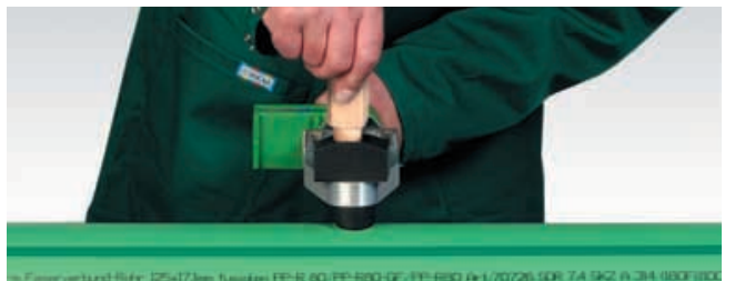
The welding tool is inserted into the pipe wall ...
