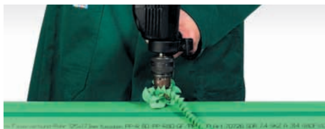
Drilling through the pipe wall
