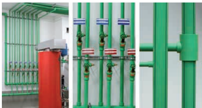
...to risers, installed with fusiotherm®-composite pipe, with conventional high rise or high rise carried out with the fusiotherm®-manifold system...
