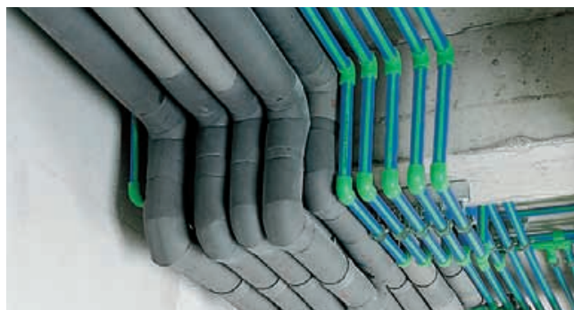
Risers and distribution piping for heating supply should be planned and installed with climatherm-faser composite pipes.
