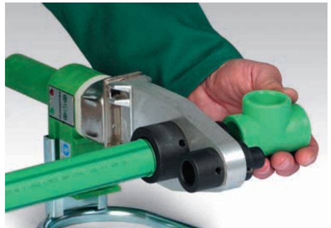
Heating-up of pipe and fitting
