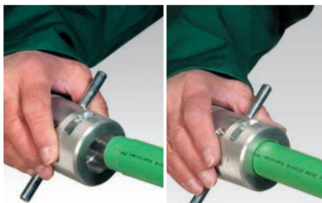
Peeling of the aluminium-PP-composite-layer respectively oxygen barrier layer (Necessary only for stabi-composite pipes and climatherm OT pipe!)
