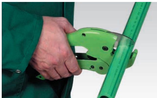
Cutting of the pipe
