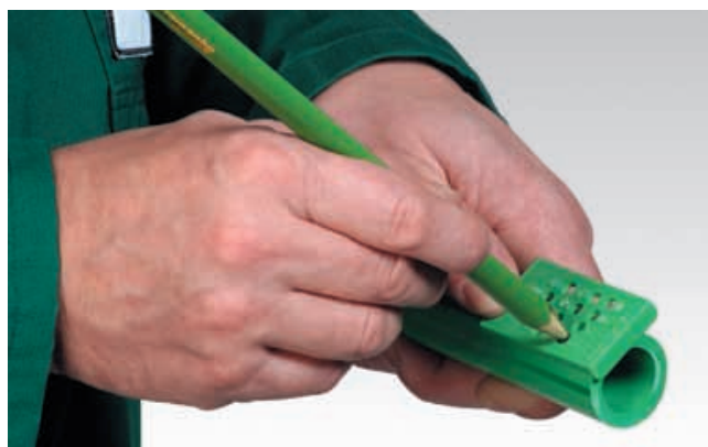
Marking of the welding depth
